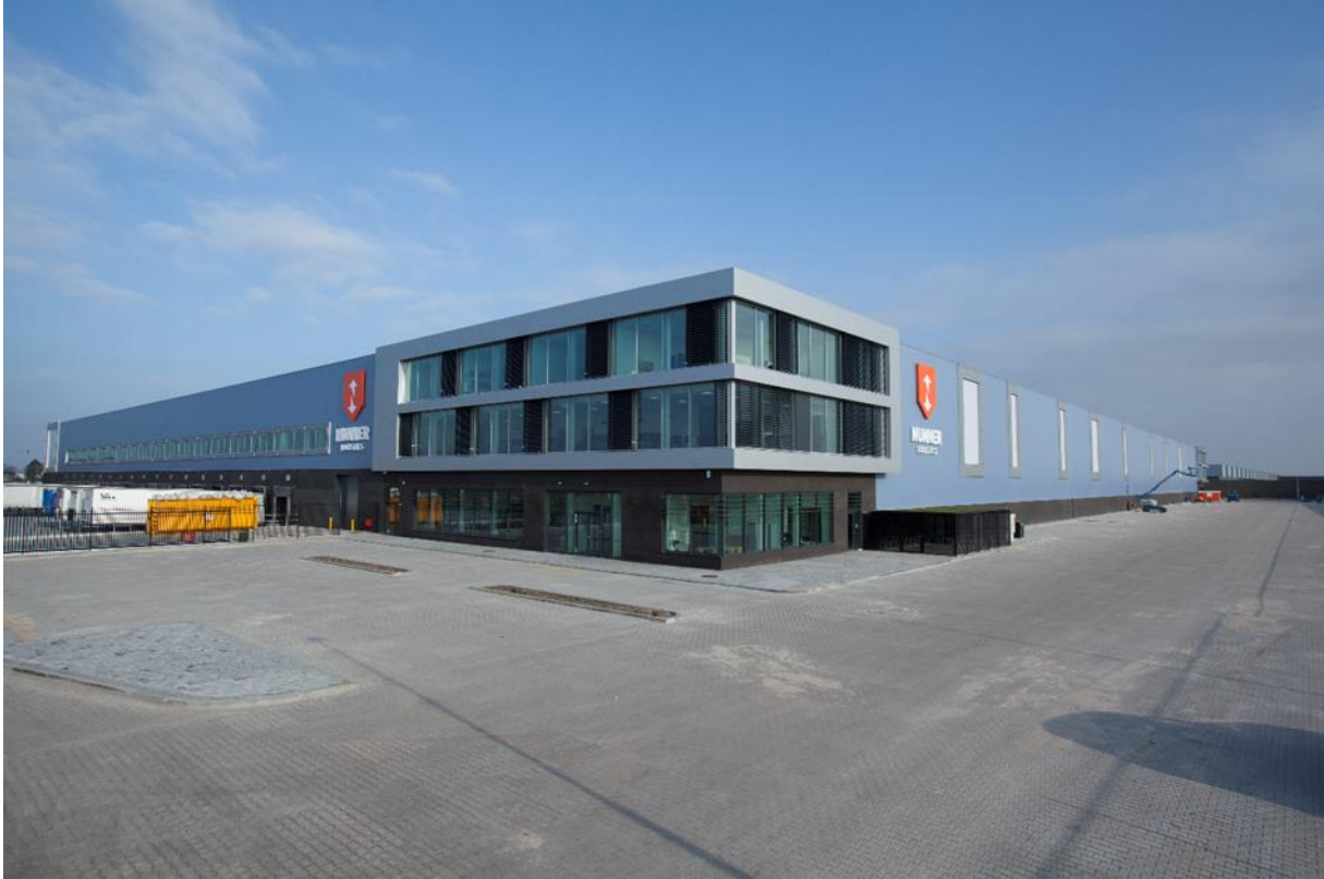
The existing site
