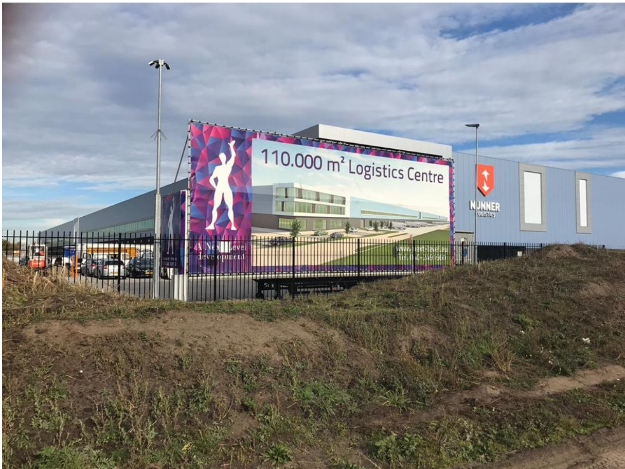
Construction sign with rendering of the expansion in front of the site
